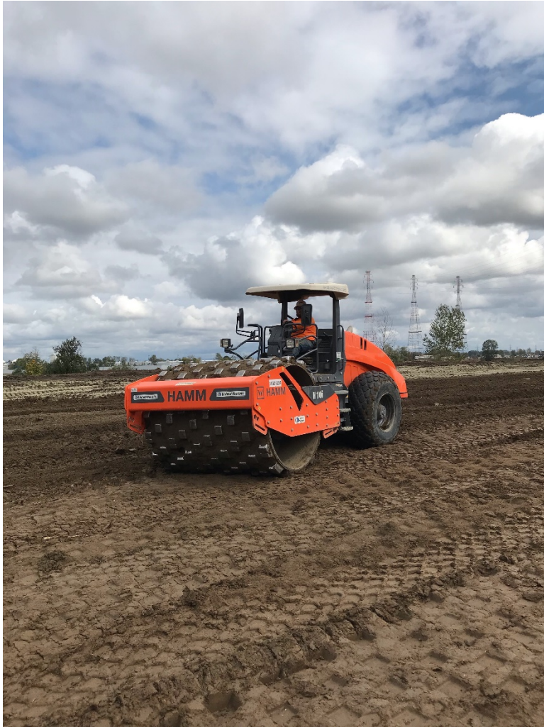
Photo 5 – Sheepfoot roller compacting soil lifts in Sub Area 2
