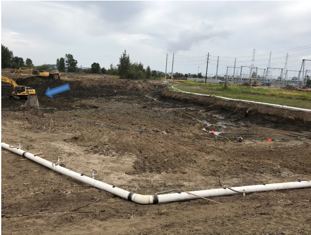
1. Photomonitoring Point 1 dewatering system and early excavation (July 7, 2020)
