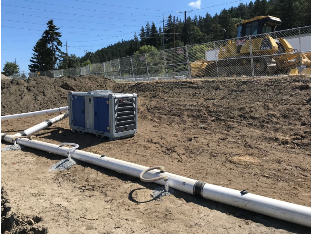
Photo 3 – Dewatering vacuum pump, collection pipe, and vertical borings
