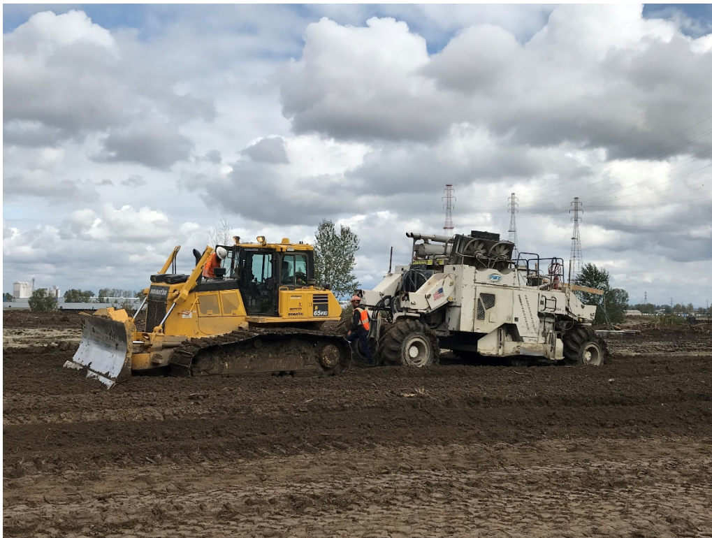
Photo 7 – Cement dust/soil mixer being extracted from soft soils in Sub Area 2.
