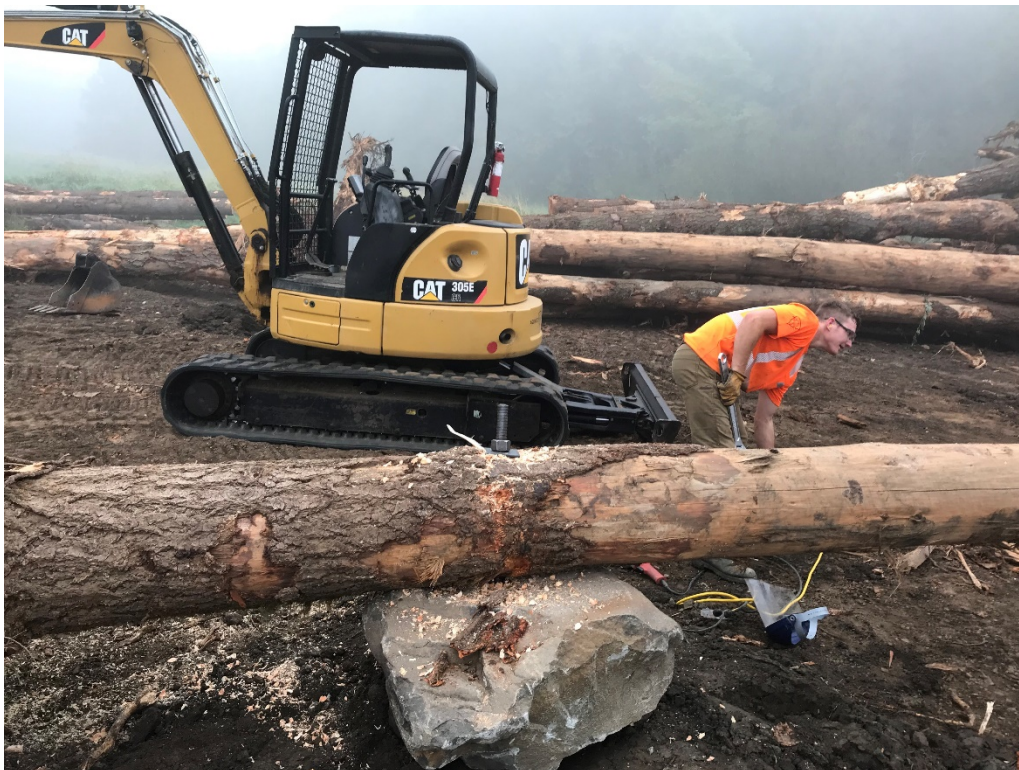
Photo 15 – Rock ballast being attached to large woody material
