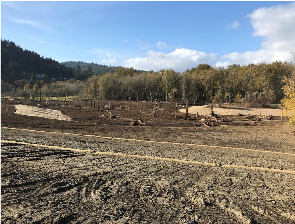
Photomonitoring Point 5 – Sub Area 2 Berm, facing northwest (Oct. 30, 2020)
