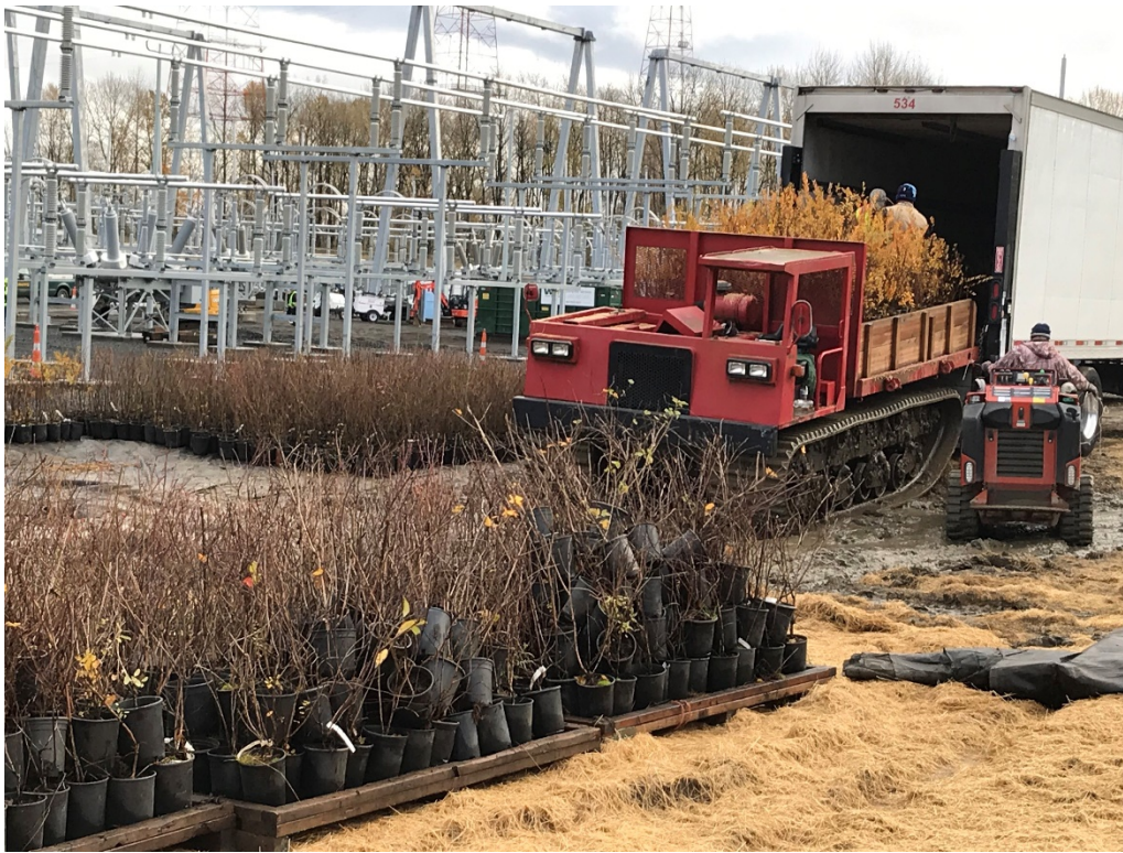
Photo 14 – Plant staging and equipment used to deliver and distribute material
