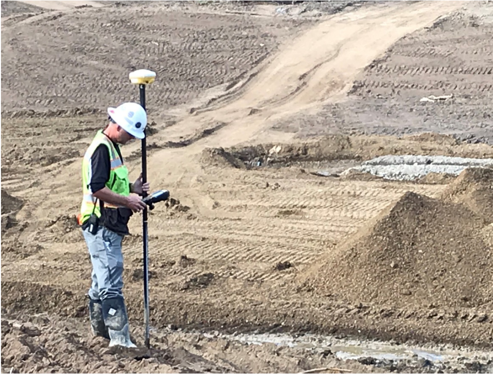
Photo 10 – Elevation spot check during construction (Oct 9, 2020)
