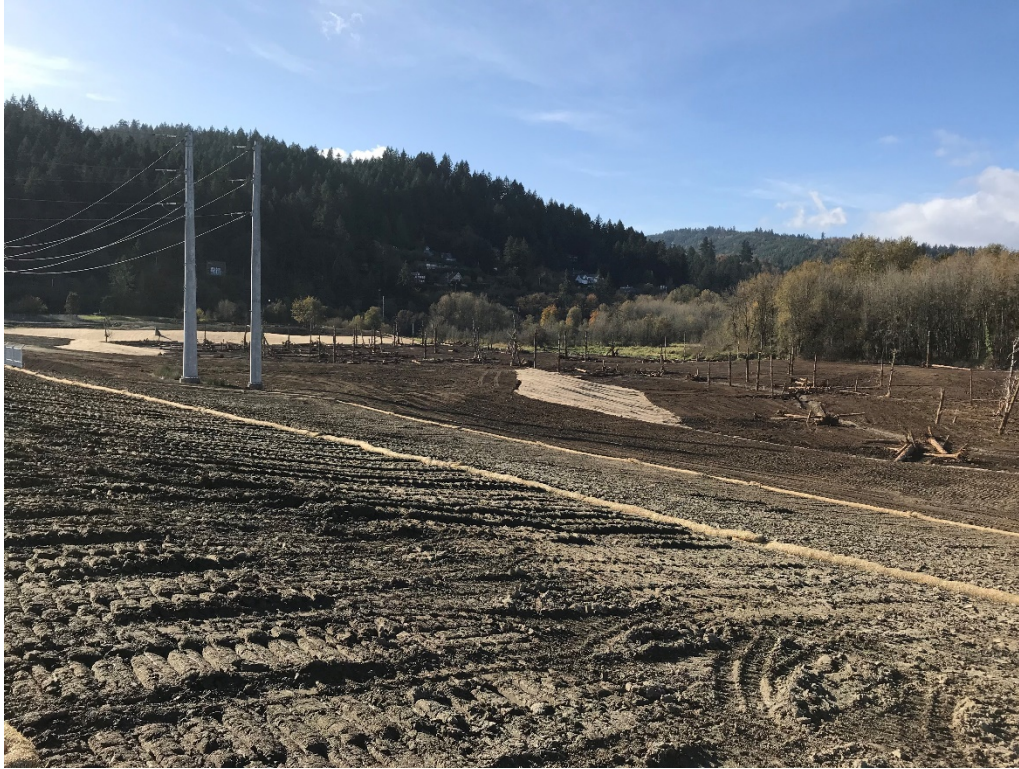
Photomonitoring Point 5 – Sub Area 2 Berm, facing west (Oct. 30, 2021)
