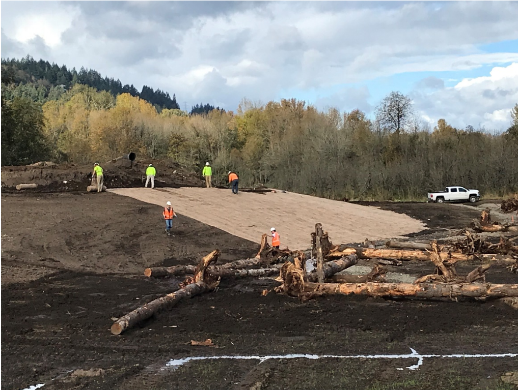
Photo 11 – Jute mat installation in Sub Area 3.
