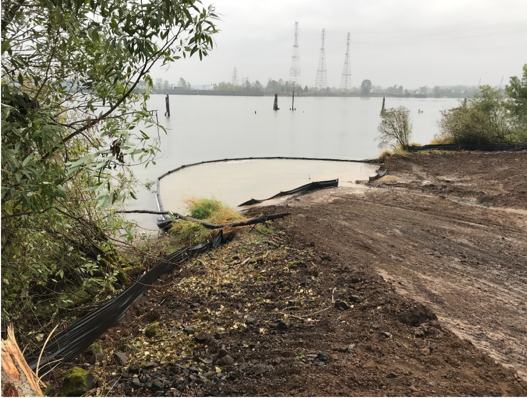
Photo 12 – Sediment curtain at the North Channel outlet (Sept. 9, 2020)
