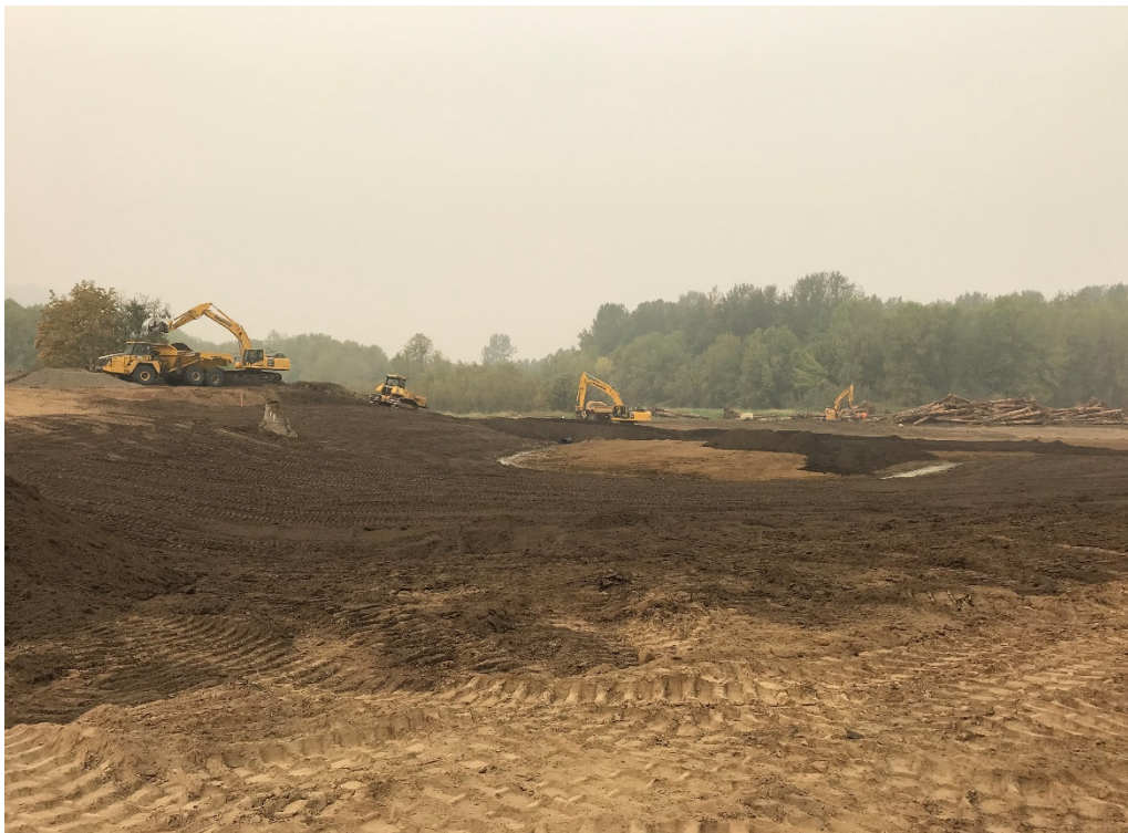
2. Storm water monument – topsoil application and early channel construction (Sept. 16, 2020)
