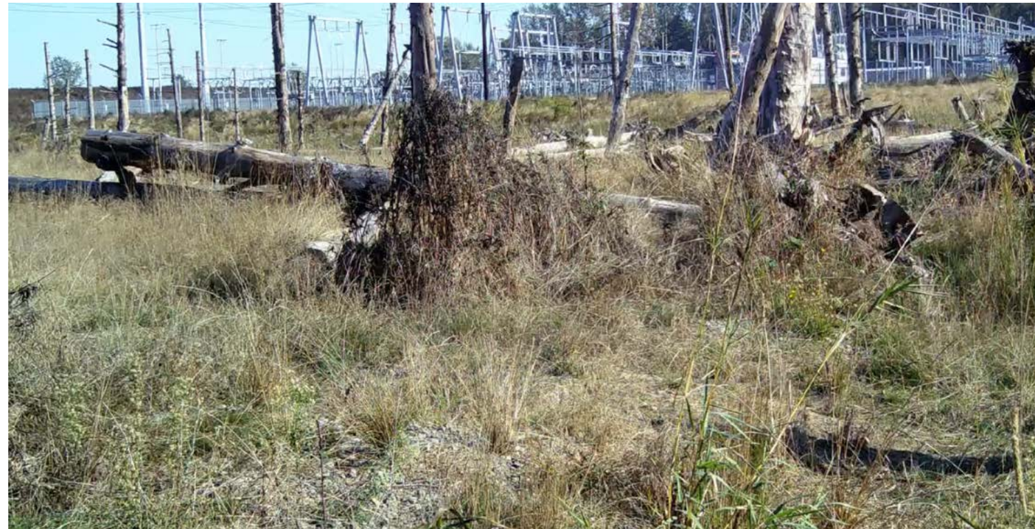
NORTH CHANNEL - PHOTO FACING DOWNSTREAM (OCT. 3, 2022)
