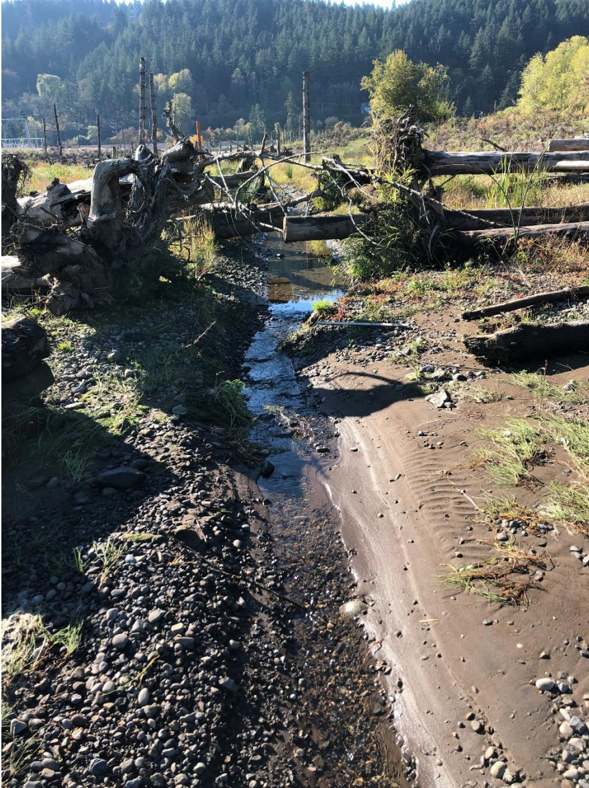
Channel Photo 3. Outlet of North Channel (facing upstream) following September rain event. Note channel morphology – loss of channel sinuosity and erosion/transport of the gravel bar formed in July/August (see Photo 2.)
