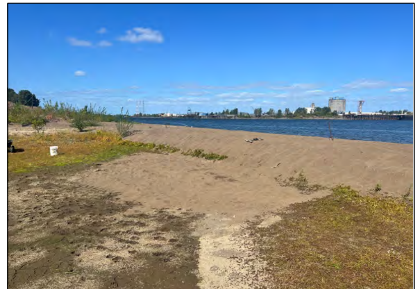
Photo 2 – Filled ponded area in OCH facing north
