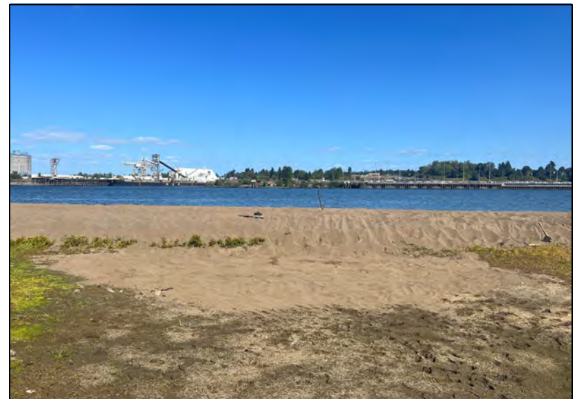
Photo 8 – Filled ponded area in OCH facing east
